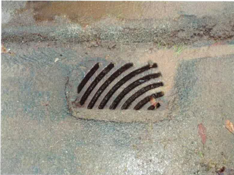
Photo 14 Storm drains are the main pathways for pollutants from road runoff to enter a stream. This was from the June rainstorm at landscape site.
