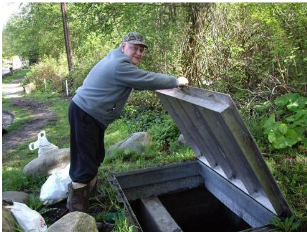
Photo 16 An oil – grit separator near Site 1, provides some treatment of road runoff in commercial and industrial area. These structures require periodic maintenance to remove accumulated oil and sediment.
